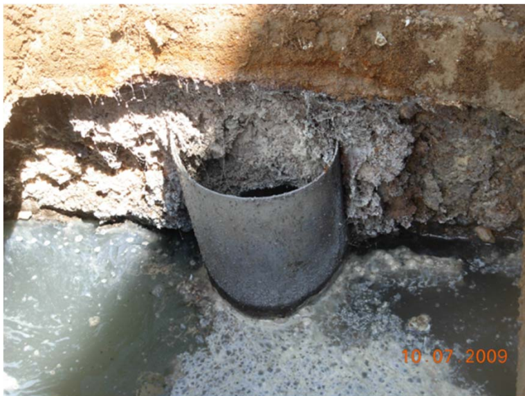
Concrete Corrosion
